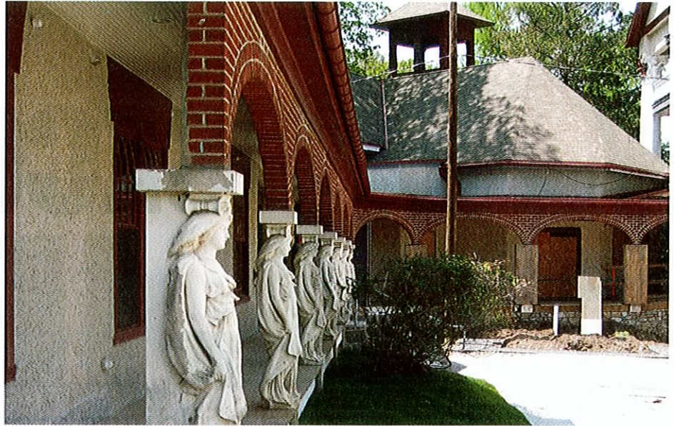
ICONIC COLUMNS: Original statuary will continue to serve as structural elements or as outdoor sculptures.
